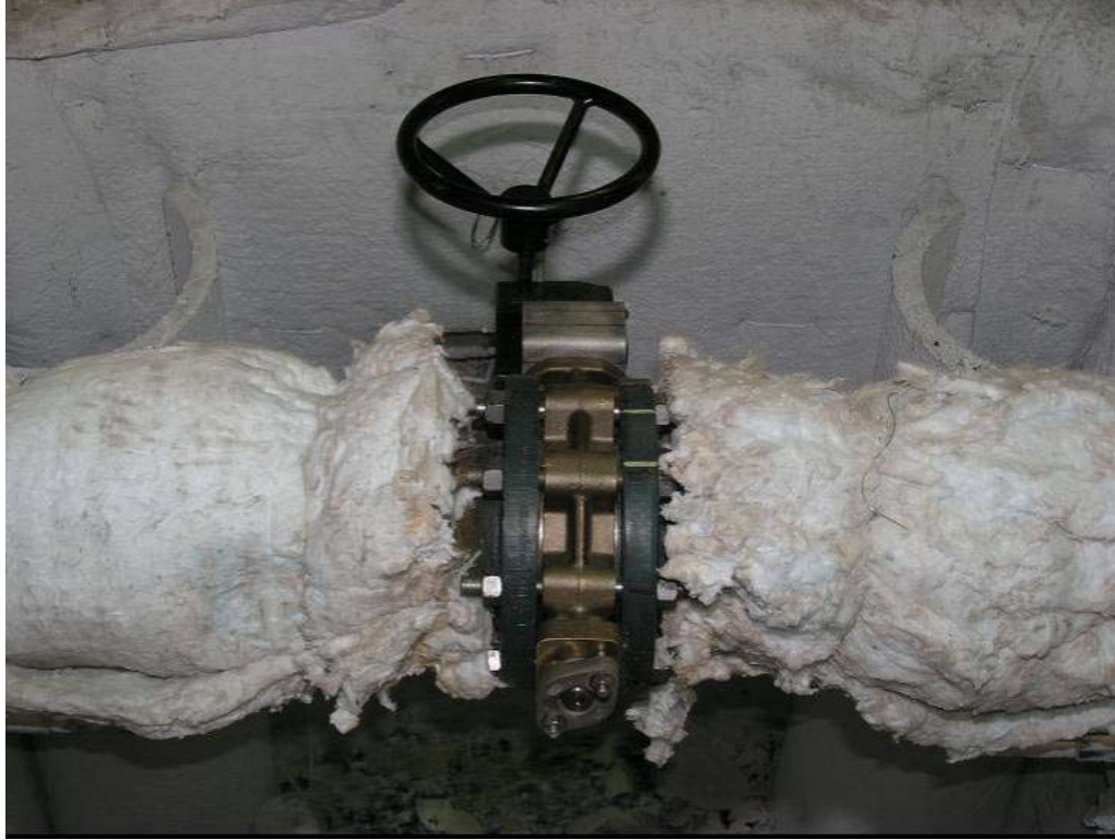
Figure A-3. 4-in. Valve in Furnace Prior to Fire Test.
