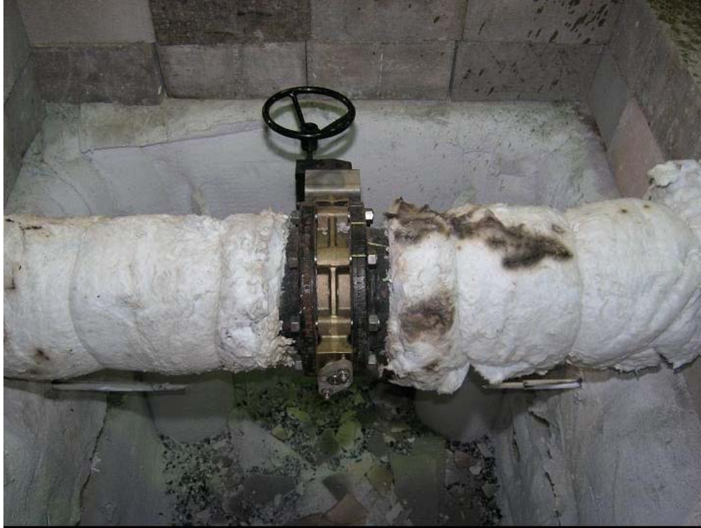
Figure A-1. 8-in. Valve in Furnace Prior to Fire Test.
